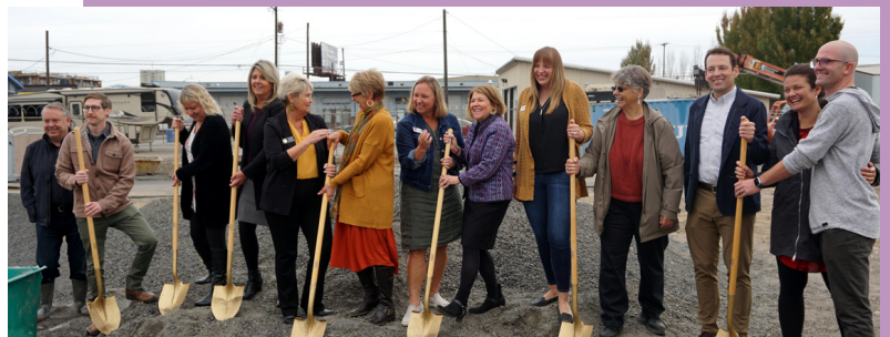
Crosswalk Groundbreaking in October 2023
